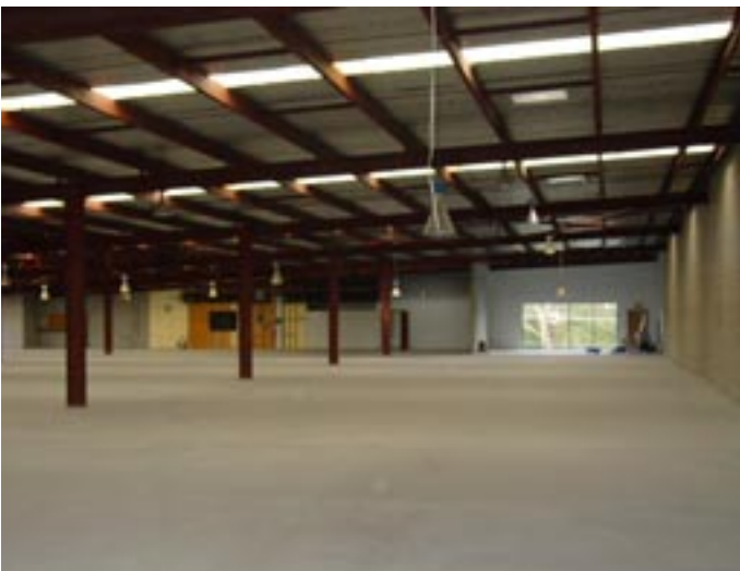
Work is just beginning on the Navman project
